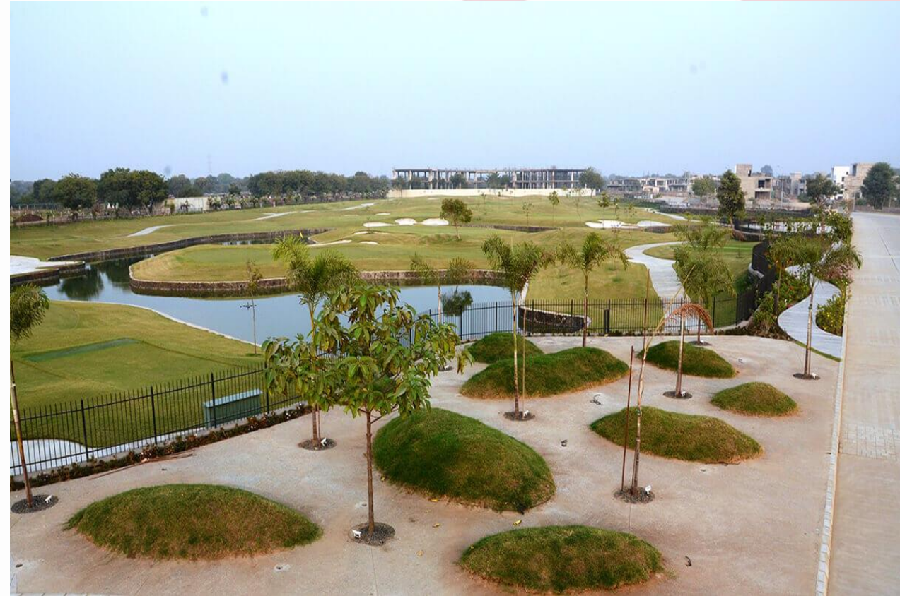
Golf Course Construction
