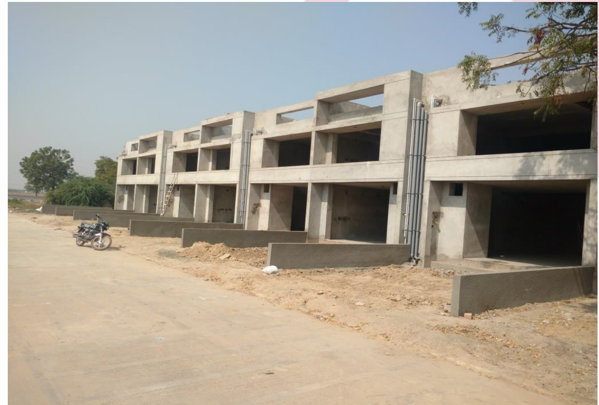
Construction work at Site
