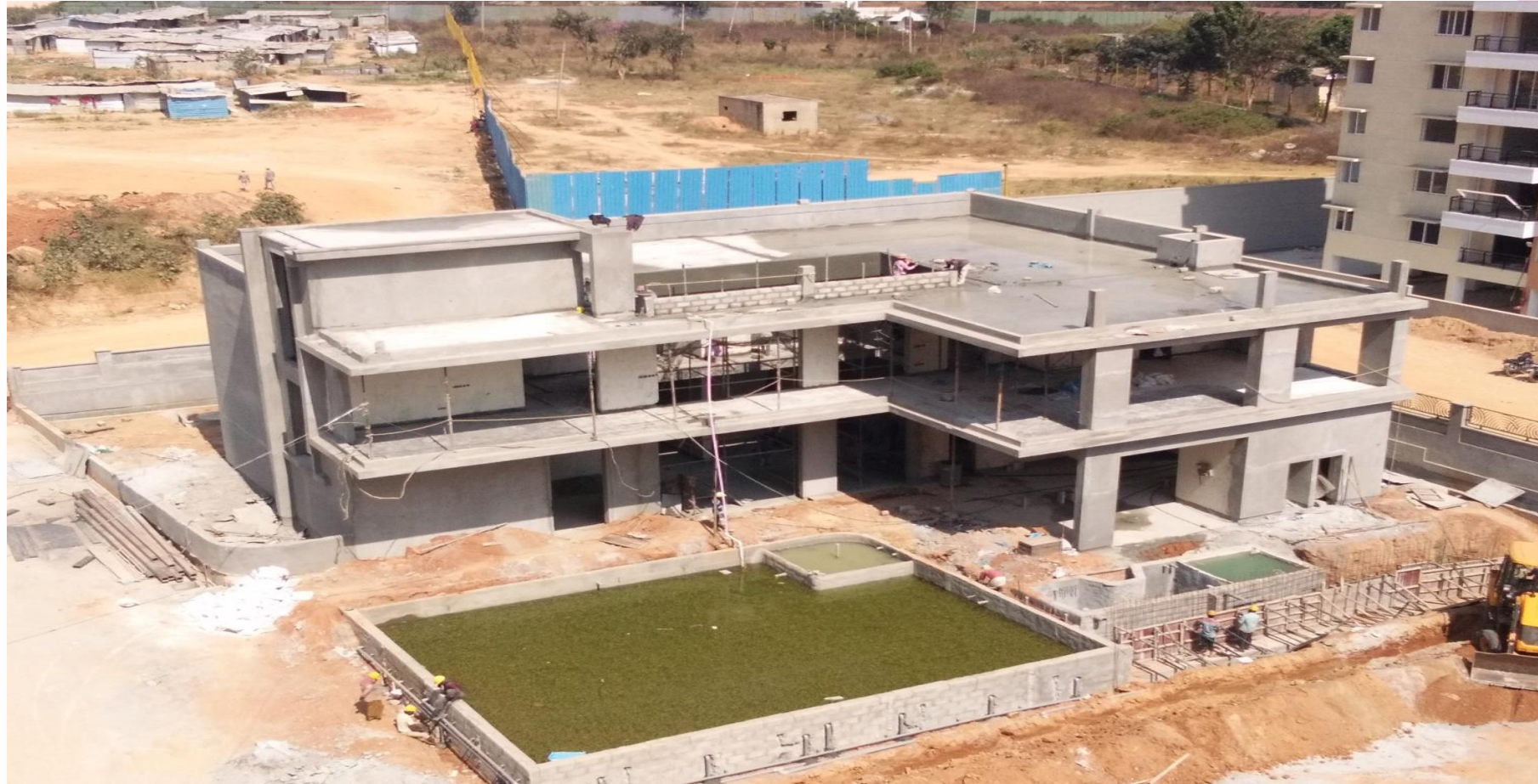
Club House Construction
