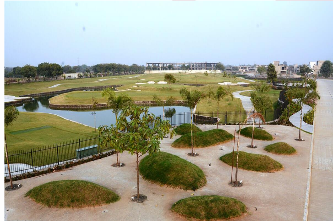
Golf Course Construction
