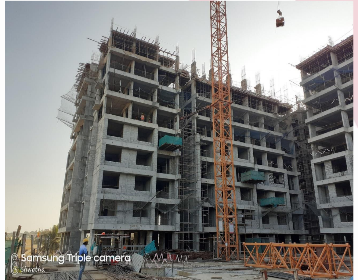
Construction at Site
