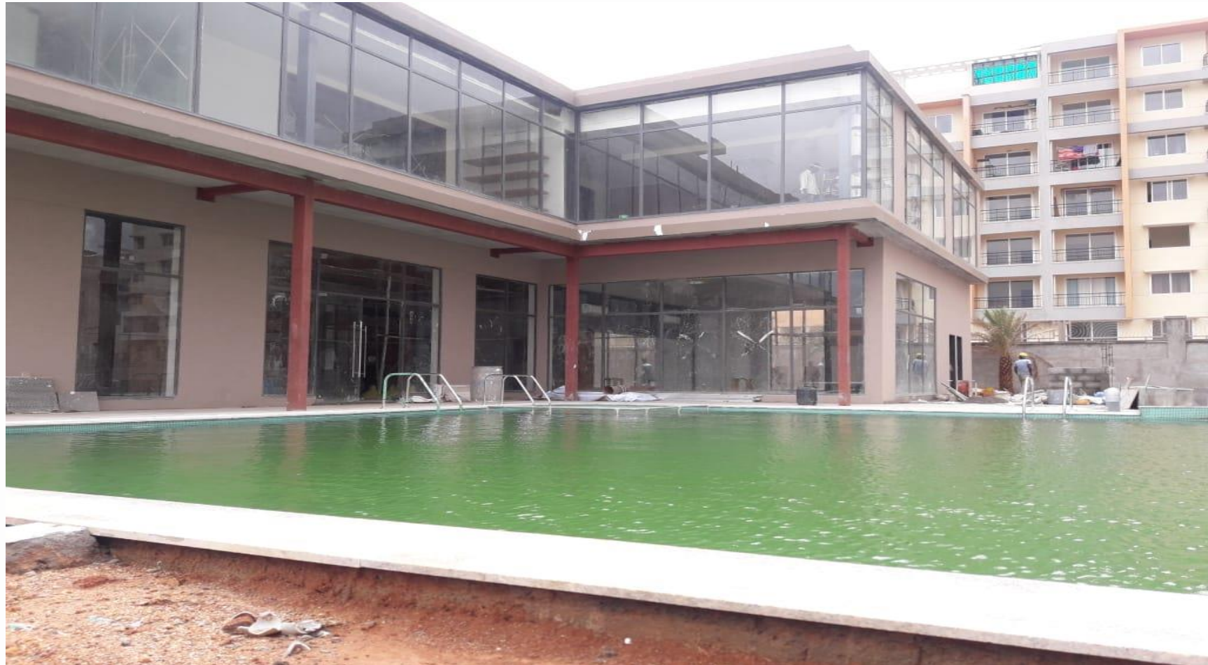
Club House Construction
