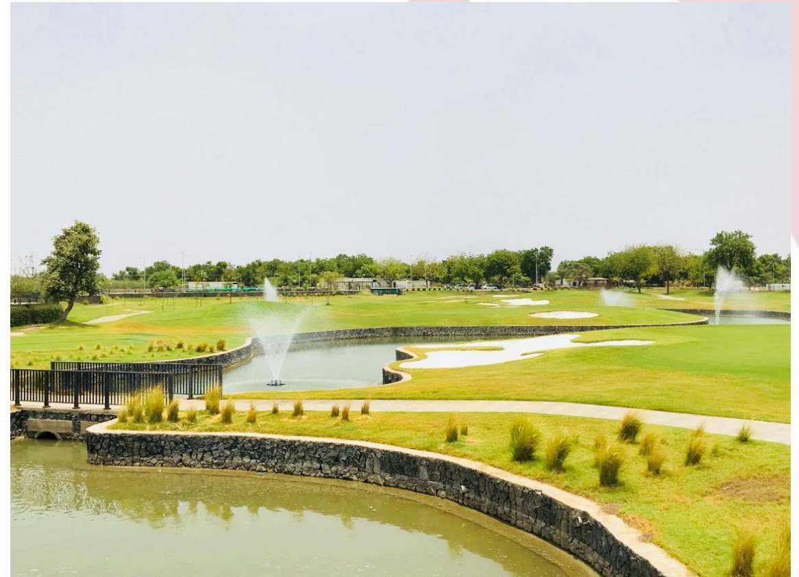
Golf Course Construction
