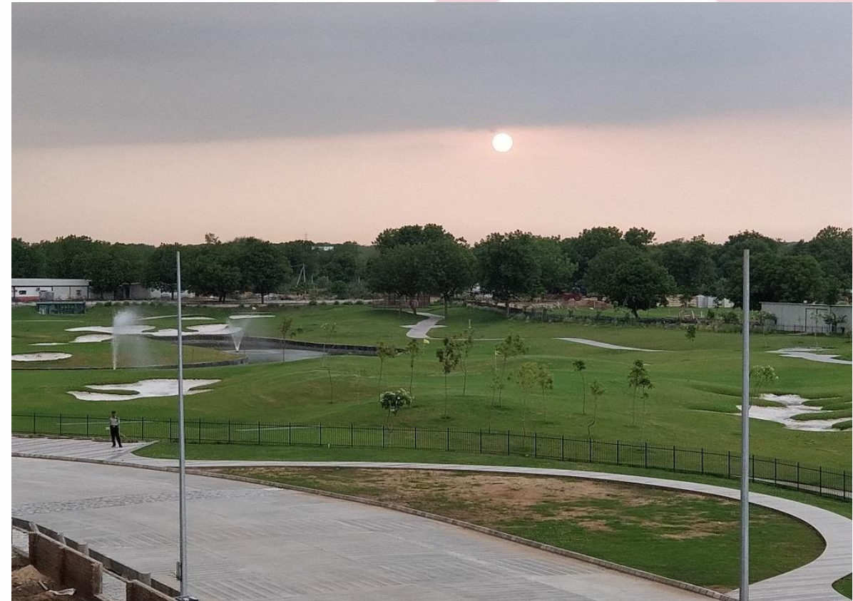
Golf Course Construction
