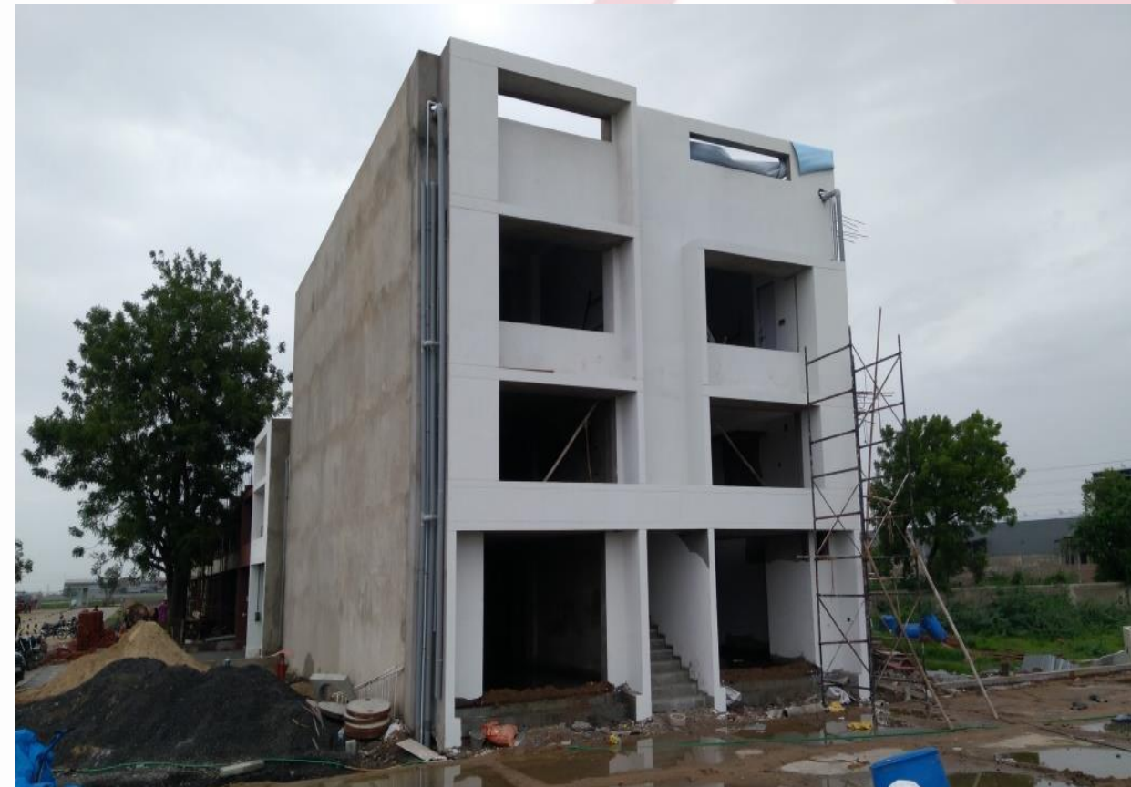
Construction work at Site
