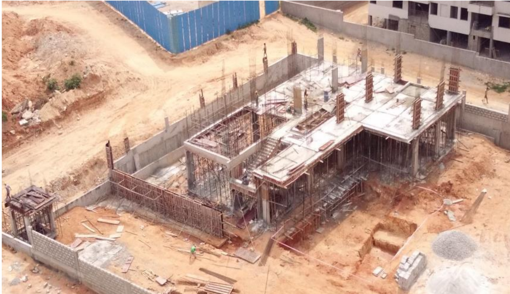
Club House Construction
