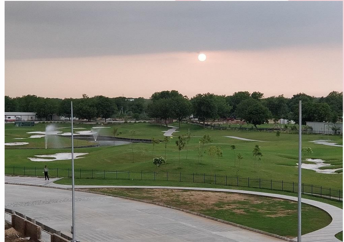
Golf Course Construction
