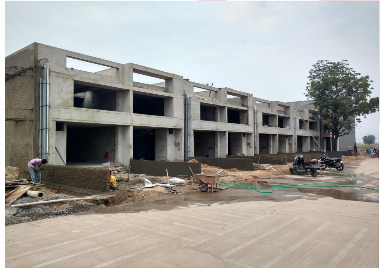
Construction work at Site
