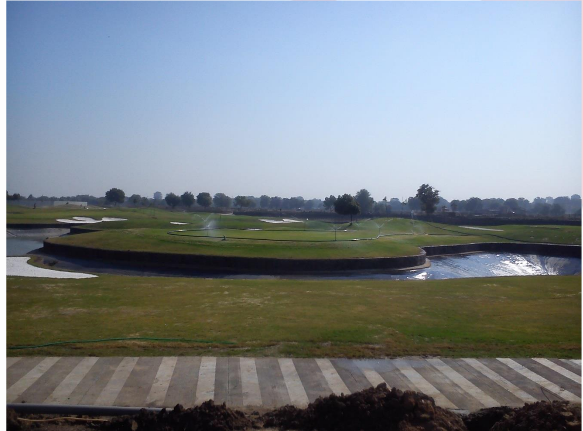
Golf Course Construction
